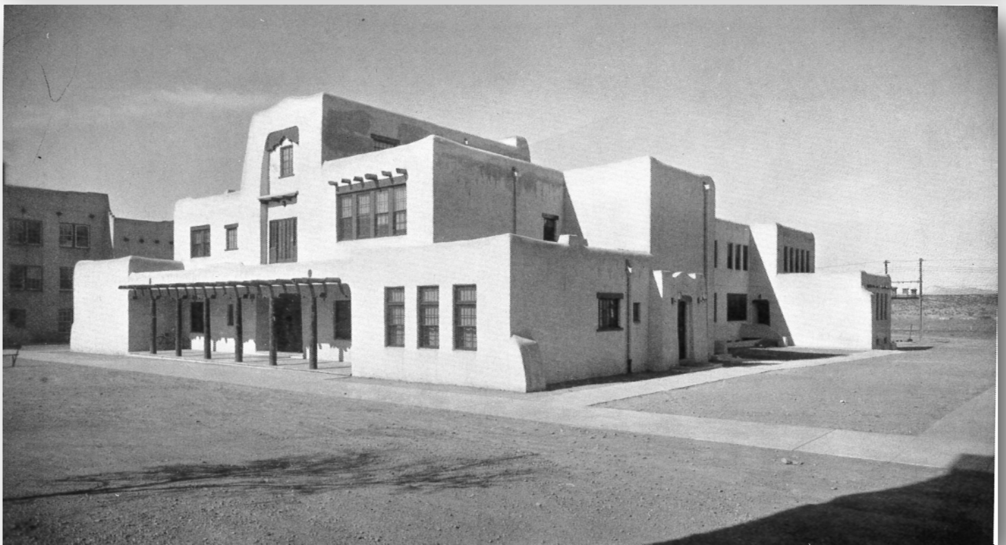
1935-36 Class/Administration Building Gordon F. Street Renamed Dillon Hall
