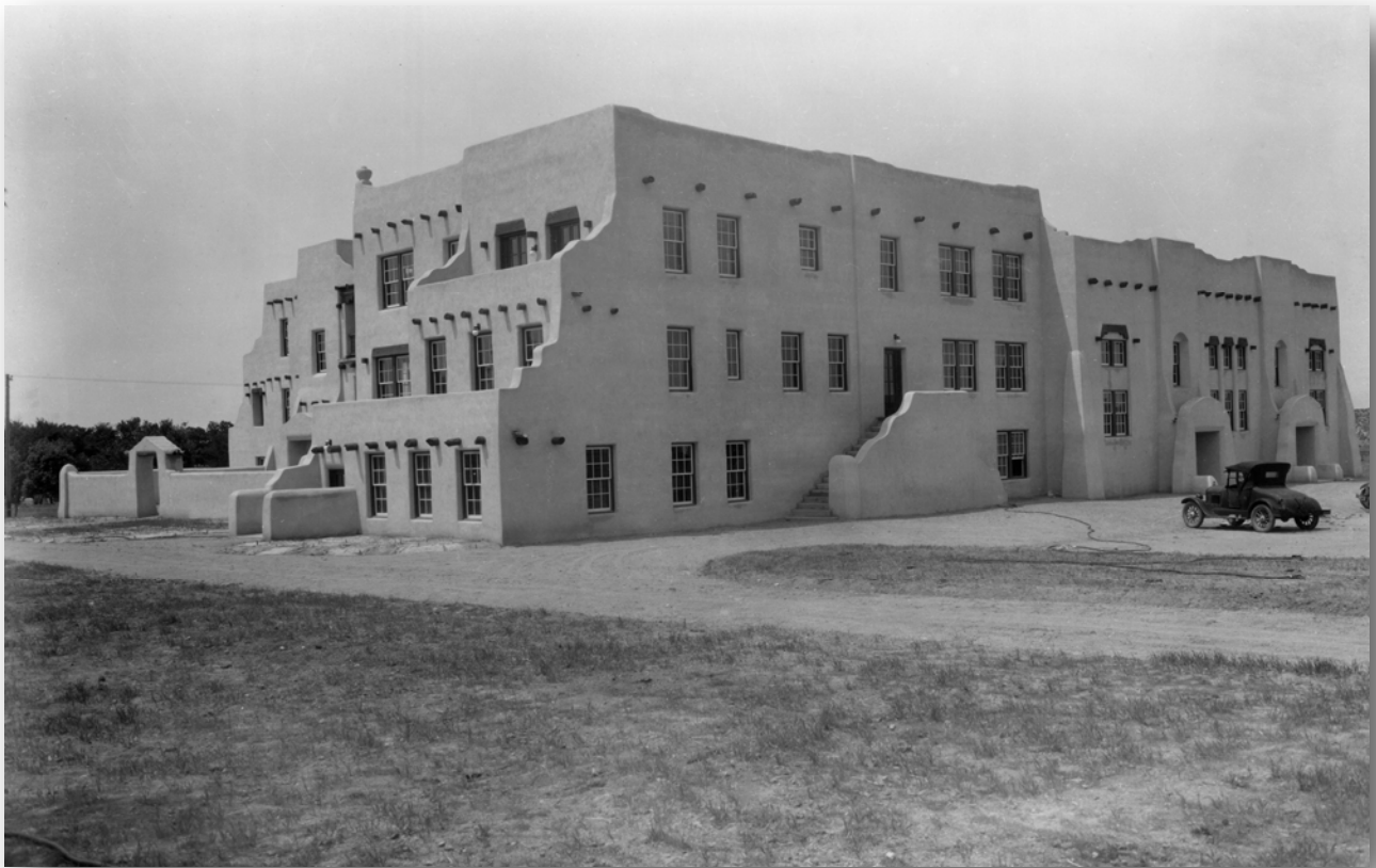
1928 Boys' Dormitory George Williamson Connor Hall
